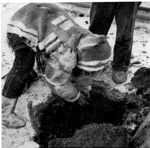
1. The "mudder" chops the moist earth fine with his snowknife (left) and takes a ball of mud . . .
